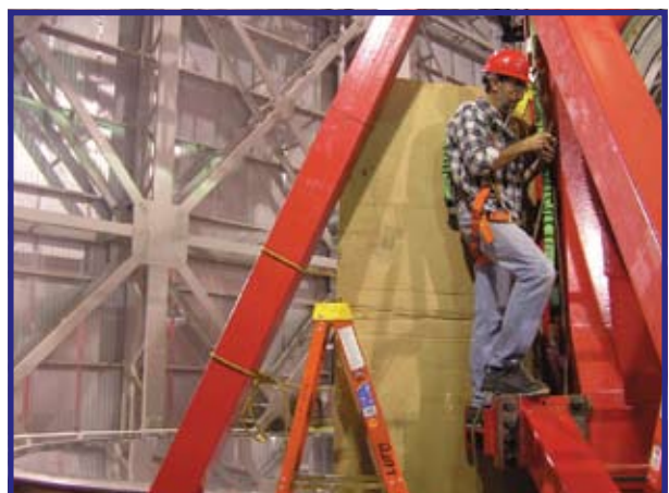
Fig. 6: Emil Popov mounts the brackets of the Permanent Fiber Focus Units to the telescope in 2007.
