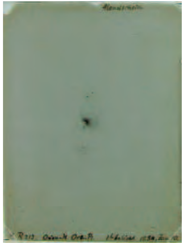
The Fig. shows one of the oldest photographic plates – a 60 min exposure of Orion Nebula, observed by Lohse on January, 10th, in 1889. Lohse used a 13 cm heliographic objective with 1.36 m focal length and 152"/mm scale, attached to the 30 cm refractor on Telegrafenberg, which was called "Großer Refraktor" in the period of 1879 -1899, before the 80 cm refractor was mounted.
